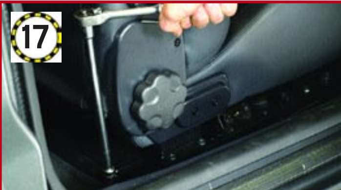
17 Tilt the seat forwards and locate the Torx T30 bolts to mount the rear of the runners. Check no additional carpet gets trapped. Don't fully tighten the bolts
